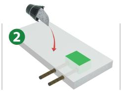
Pouring concrete around the Rezaboite P. The ducts are protected.
